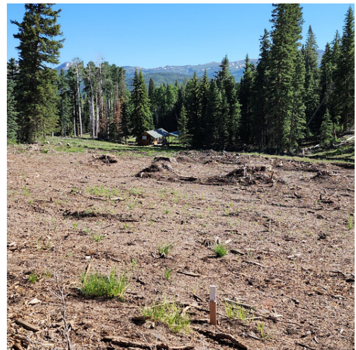
Lead-contaminated soil was neutralized and moved to an approved off-site facility.
